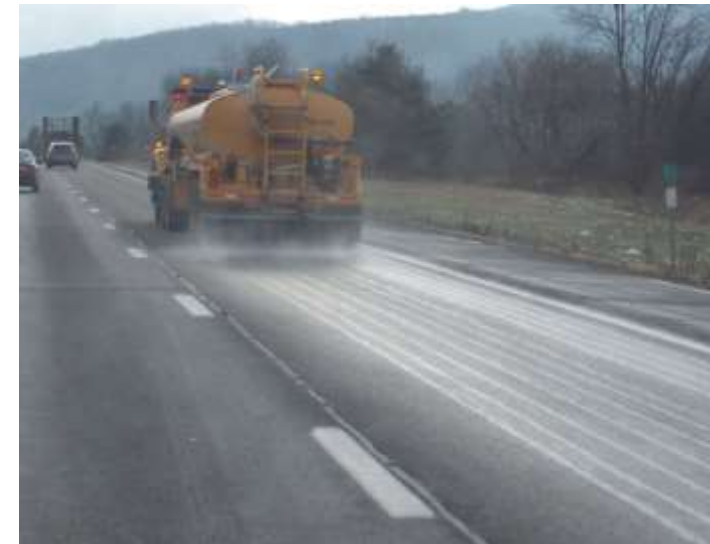
Anti-Icing the road before the storm
