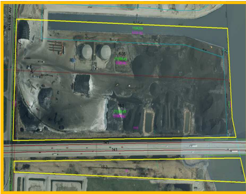
Aerial of Fox River Dock Company Incorporated, Port of Green Bay, WI.
