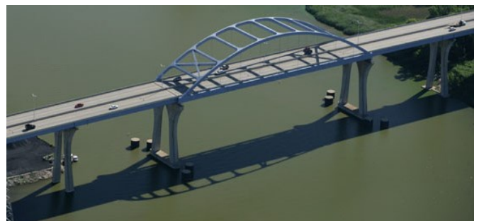
Leo Frigo Bridge has 119 Feet Vertical Clearance
