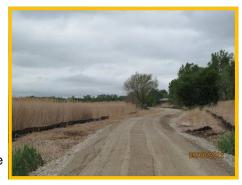
tions. Twelve of the tests were in the compacted area of the road and exceeded the specifications requirements of 95% compaction. Two tests completed in the center of the road where no wheel traffic occurs were 90 and 91%, but are not of significant concern as no wheel traffic will occur on the center of the road.
