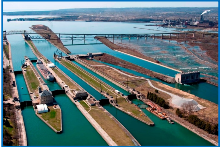
Credit: USACE. Soo Locks Image
