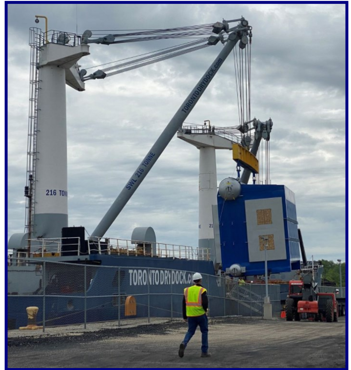
A 200 ton boiler being lowered at the Georgia Pacific plant in Green Bay on Jan 1, 2020; Credit: WLUK
