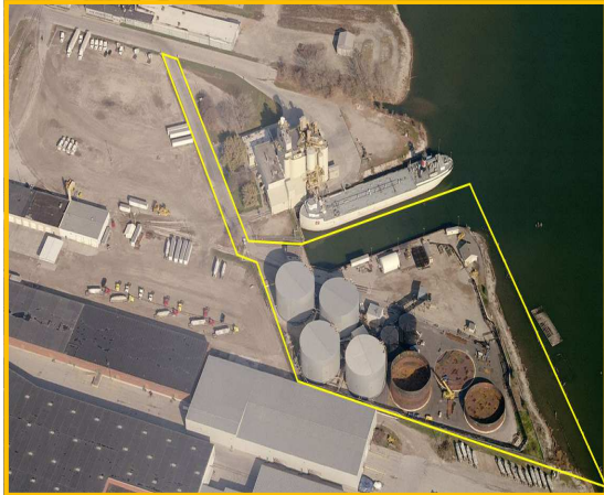
Aerial of Construction Resource Management on the Fox River, Port of Green Bay, WI
