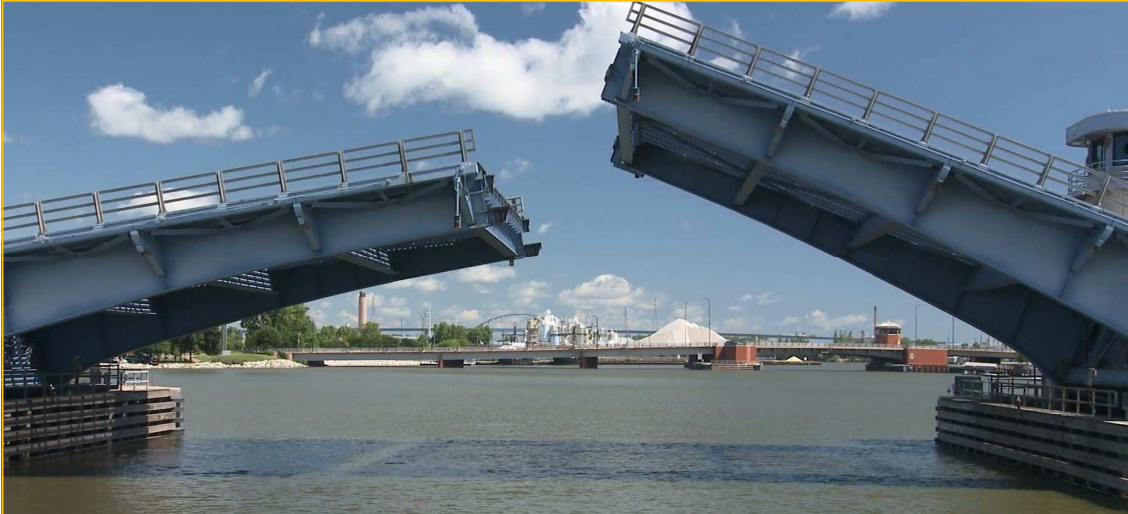
Walnut St. Bridge looking north to Main Street
